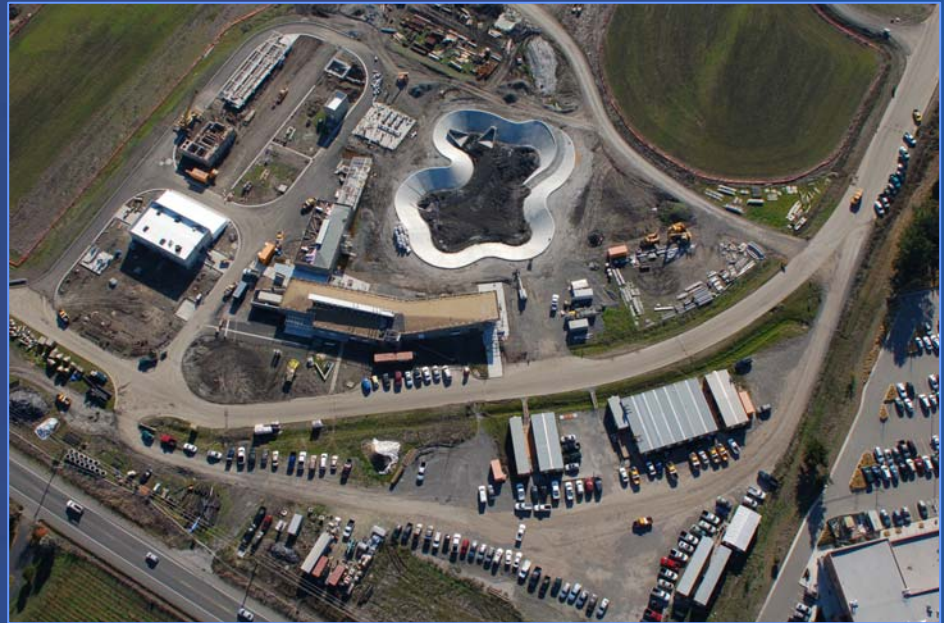
Tertiary treatment area of the Ellis Creek Water Recycling Facility
